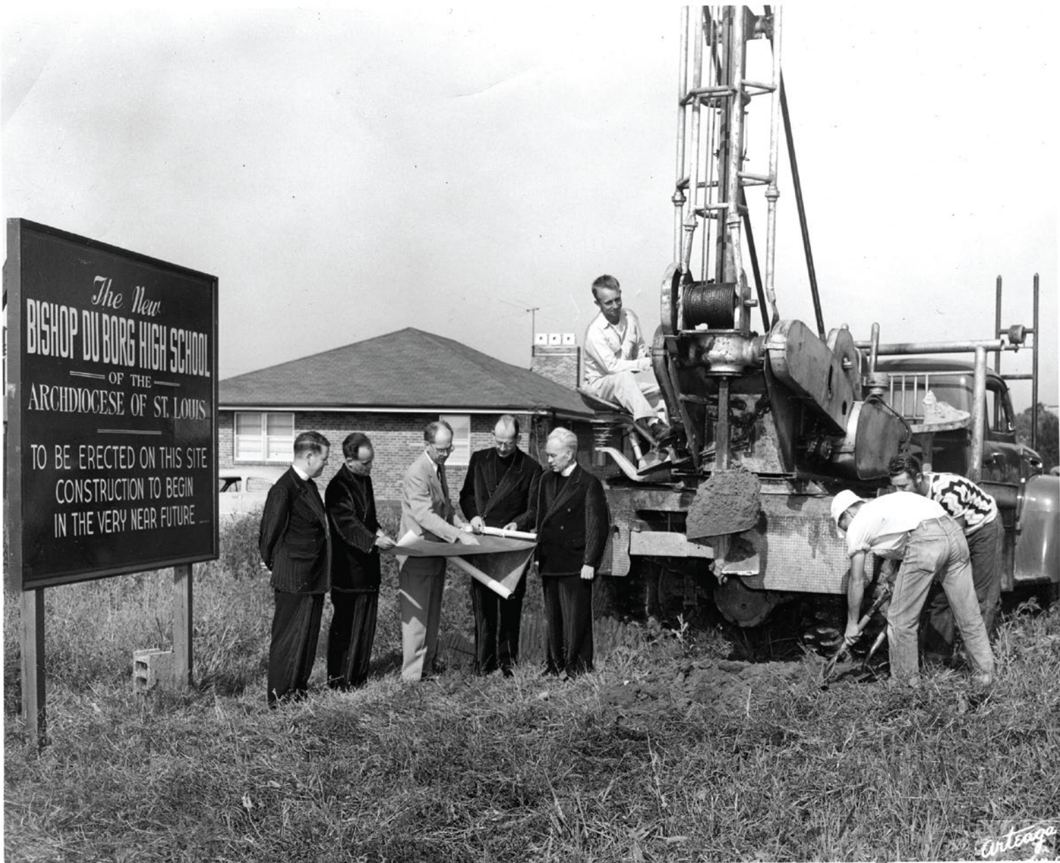
Bishop DuBourg High School construction, August 17, 1951
